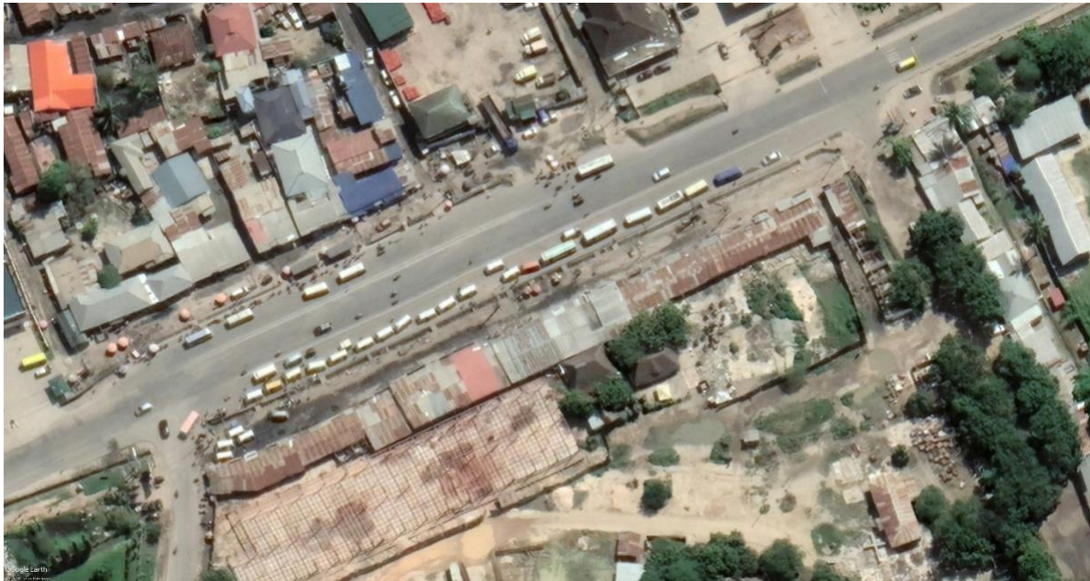
Figure 9.2-4: Bus bays at Ukonga Banana, Dar es Salaam
