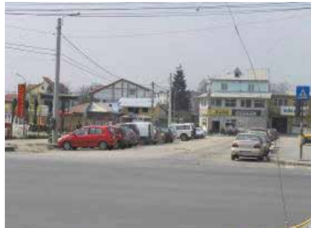
THE MIX OF PARKING PLACES AND INTERSECTION IS NOT ARRANGED SAFELY AT STREET SECUIOR
