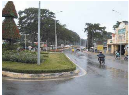
JUNCTION AT KM234 UNSAFE JUNCTION DESIGN, INSUFFICIENT TRAFFIC SIGNINGS, THE SIGHT IS OBSTRUCTED
