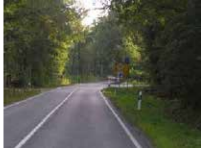
FIGURE 2 – Y-TYPE INTERSECTIONS (LEFT) AND INTERSECTION OBSCURED BY VEGETATION
