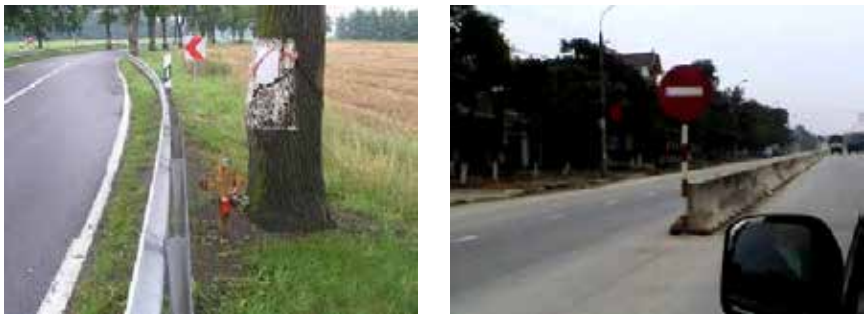
FIGURE 5 – BARRIERS IN FRONT OF HAZARDS
