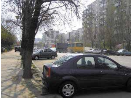
URBAN DISTRIBUTOR ROAD WITH 4 LANES AND UNSAFE PERPENDICULAR PARKING ON BOTH SIDES
