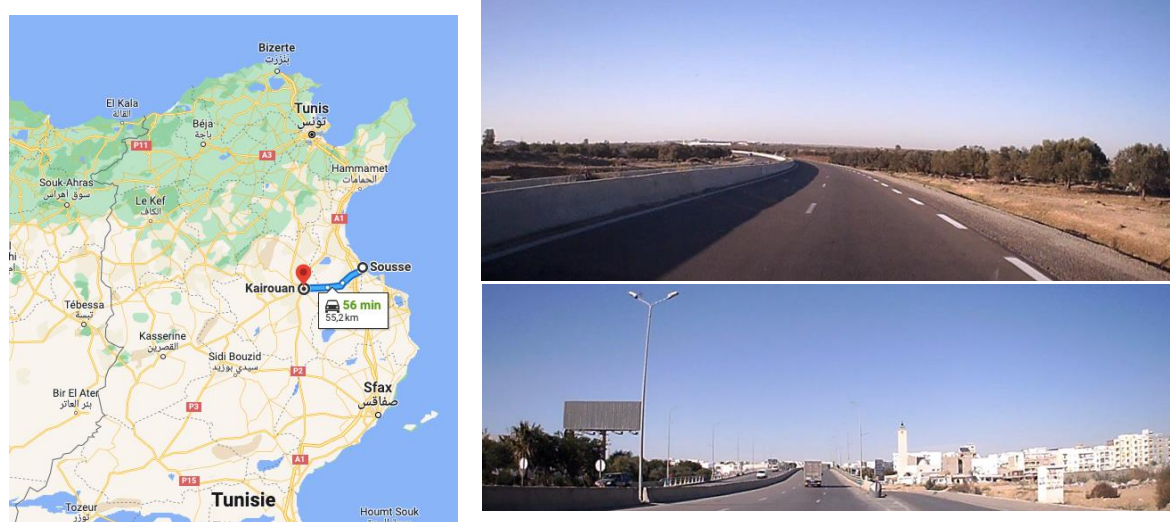
Figure 8 - Left: N12 road between Sousse and Kairouan, right: cross sections after works
