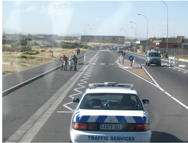
Illustration 57: Use of bottleneck and optical illusions in South Africa to instruct the pedestrian walk and to re-duce speed [9]
