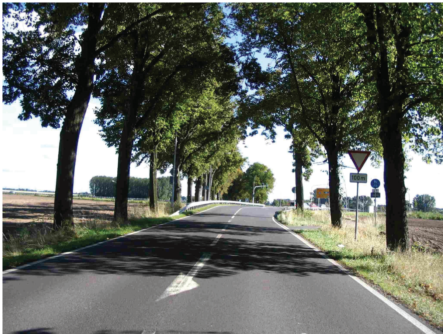
Illustration 60: Changed road direction is not unambiguously visible, the anticipation of the road course is disturbed. [12]
