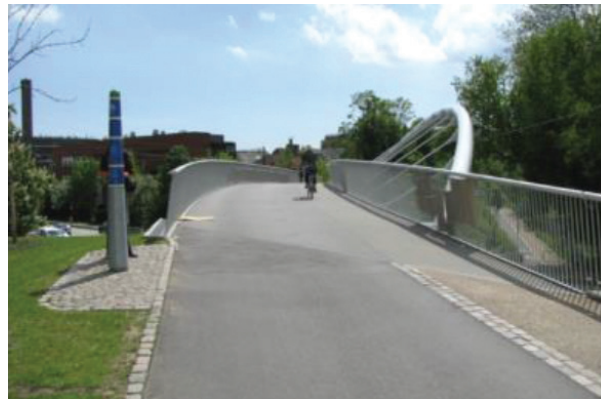
Illustration 24: Destabilisation by a non-orthogonal and unsymmetrical suspension: balance is disturbed and field-dependent users tend to swerve to the right [18]
