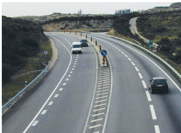
Illustration 68: Three critical locations on the left lane: end of acceleration lane, end of climbing lane and end of intersection's median. (C. de Almeida Roque)
