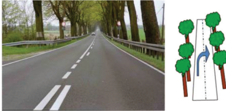
Illustration 23: Destabilisation by non-orthogonal impression: field-dependent drivers spontaneously swerve and cause accidents [13]
