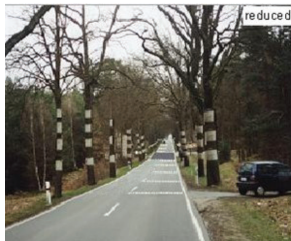
Illustration 7: Improved situation by optical countermeasures of space perception (simulation) [7]
