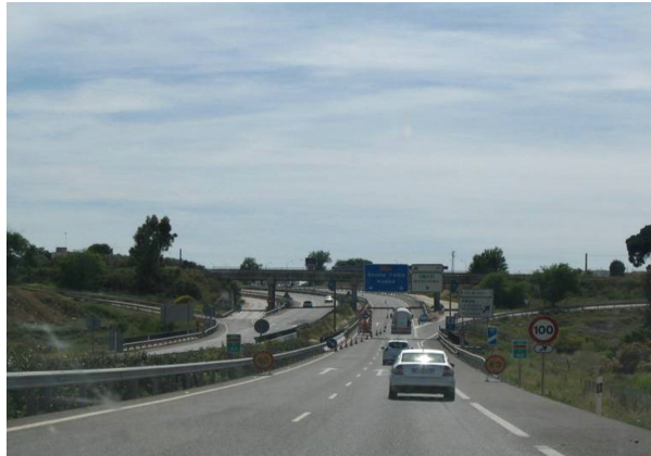
Illustration 67: Three critical locations: maintenance location, starting a curve and exit road without transition and/or progressive information (150 m ahead). [12]
