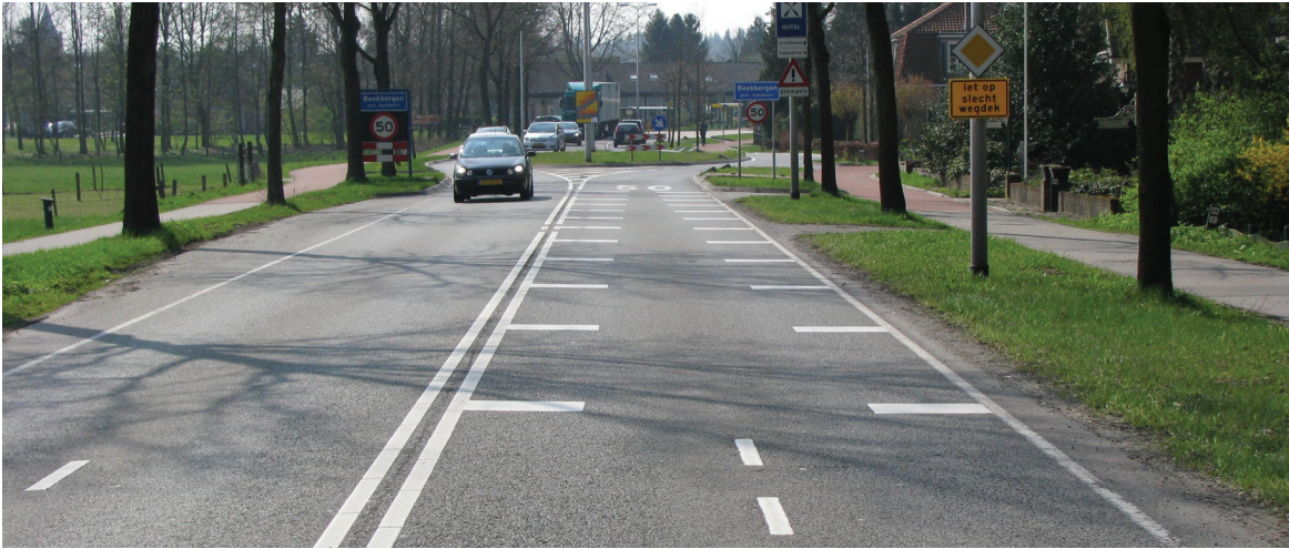
Illustration 85: Town entrance combined with a middle island and marking to signalise the change of driving programme [38]
