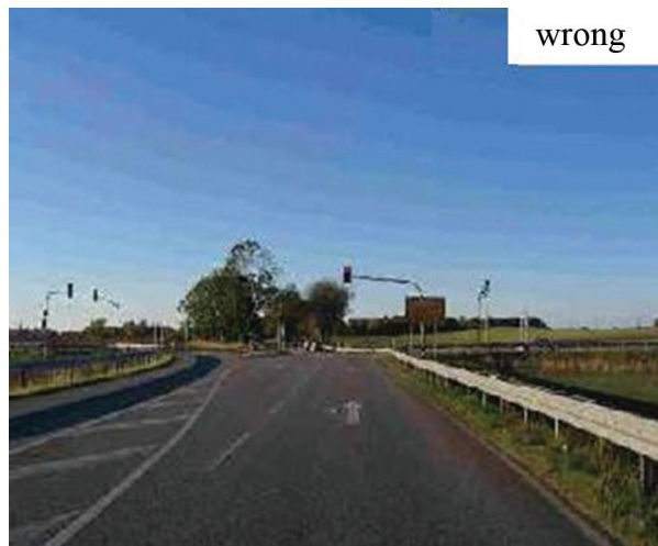
Illustration 5: Junction, perceptible only at 100 m distance: the minor road seems to be the main road; unexpected braking and high speed at this location cause rear end and sideswipe collisions [10].
