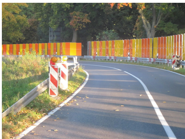
Illustration 81: After: the course of the curve has a clear guidance, the coloured setting guides the driver, sig-nalises the course and reduces speed. The alternative colours work like an optical break. [15]
