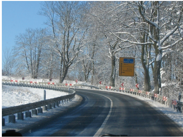
Illustration 80: Before: the course of the curve is discontinuous, drivers underestimate the radius. The speed is too high, about four fatal accidents/year. [15]
