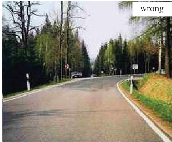
Illustration 61: Optically misleading view axis: road curves to the right contrary to the view axis leading straight ahead (150 m before the critical location). [12]
