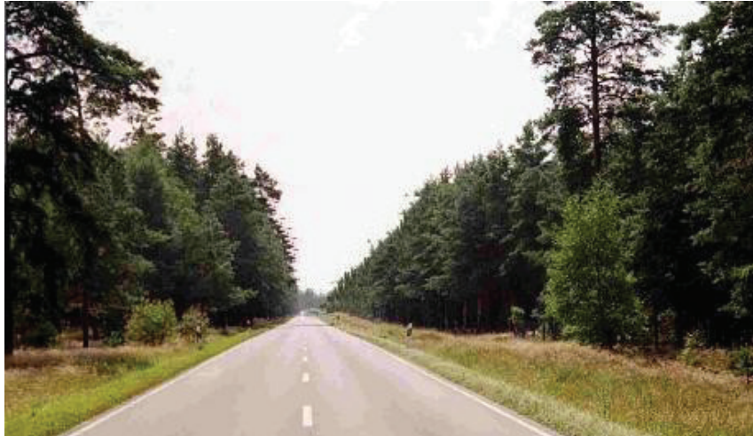
Illustration 16: Optical orientation to the horizon: distant focus and monotony decreased workload and cause sub-conscious acceleration. [13]
