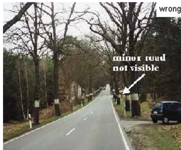
Illustration 6: Minor road is not visible early enough: unexpected braking and high speed cause rear-end collisions [7]
