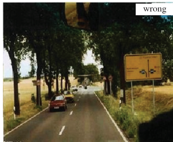
Illustration 74: Incorrect expectation of the situation caused by misleading signs at an accident location. [10]
