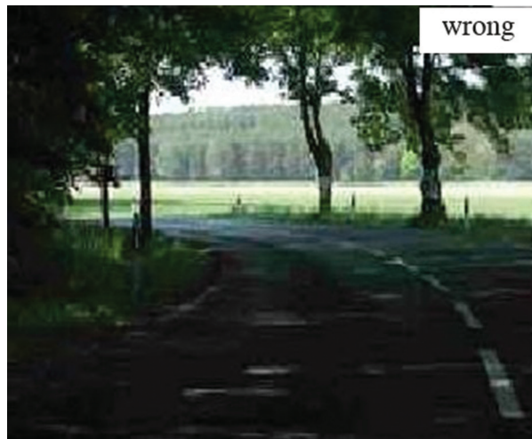
Illustration 20: Tendency towards the outer curve by misleading gaps in the setting and obstructed inner curve [12]
