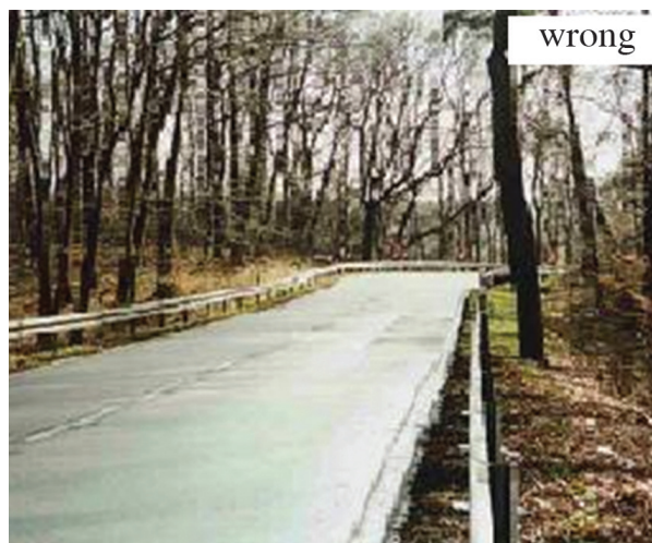
Illustration 70: Three oversized chevron signs are not visible against the background in an accident curve. [8]
