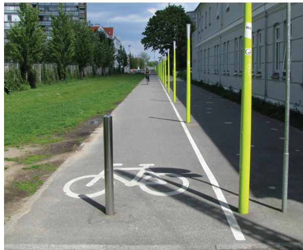
Illustration 32: Best practice example from Denmark: well-structured field of view with clear lines of reference [3]
