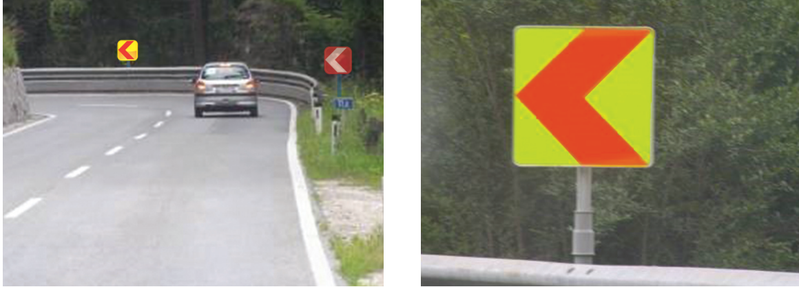
Illustration 71: Improved visibility of signs by use of yellow background instead of red. (source: photo from Austria, Hans-Joachim Vollpracht, 2008)
