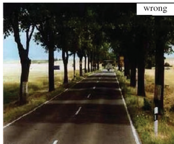
Illustration 64: Sudden change of road characteristic: the new intersection is not introduced by progressively implemented transition zone (150 m ahead). [10]
