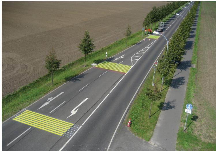
Illustration 48: Application of colored markings to guide drivers' attention to an invisible intersection (OU Forst. Source: Steffen Wenk, MIL Brandenburg, Germany)
