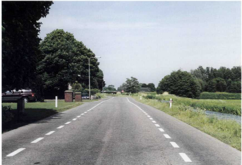
..... Figure 6.61 Cycle paths on wide 60 km/h rural road (example on urban boundary)
