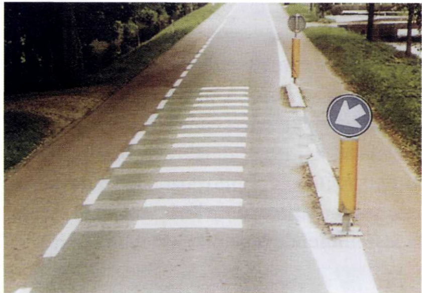
..... Figure 6.53 Threshold treatment-80 km/h rural distributor to narrow (<5m) 60 km/h rural access road
