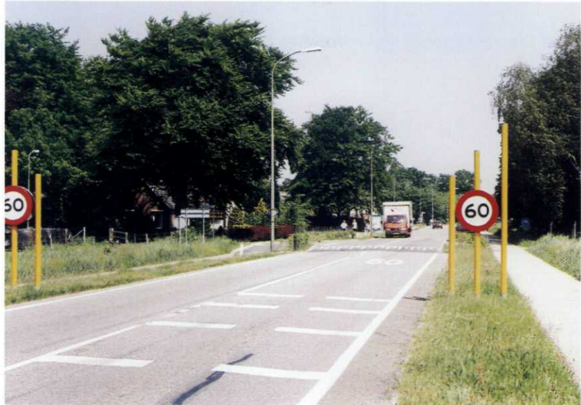
..... Figure 6.52 Threshold treatment - 80 km/h rural distributor to wide (>5m) 60 km/h rural access road
