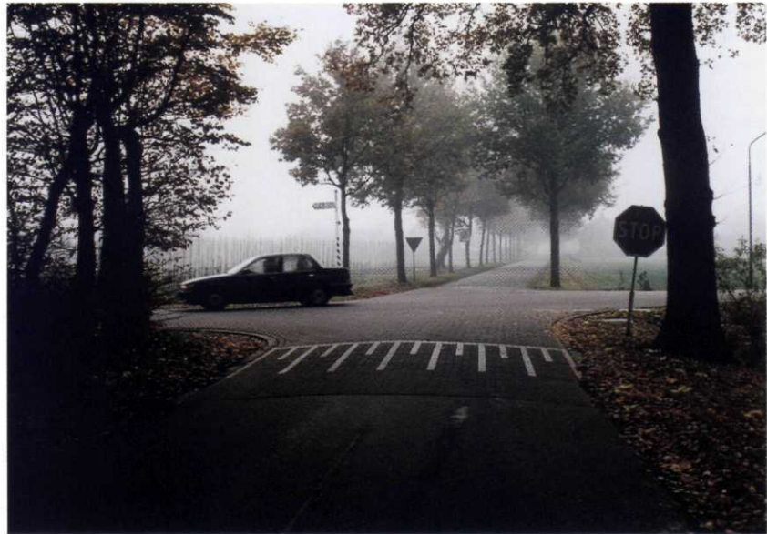
Figure 6.56 Raised intersection in 60 km/h zone
