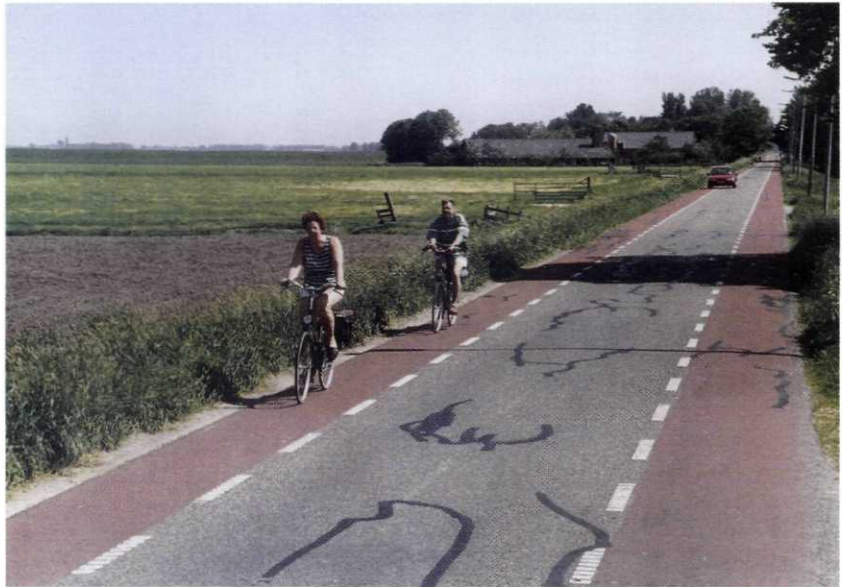
..... Figure 6.60 Narrow passing or cycle strips on 60 km/h rural road
