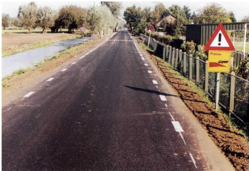
..... Figure 6.58 Edge line marking on 5 m wide rural access road
