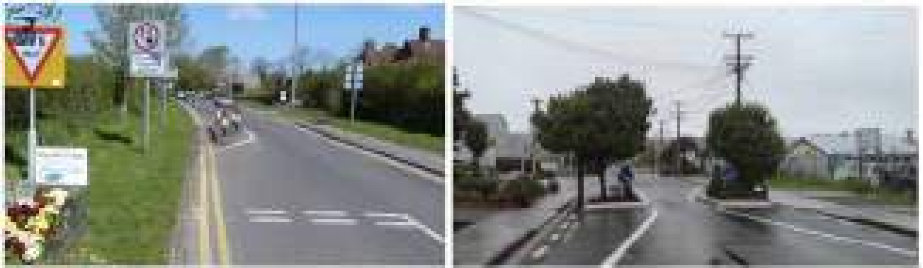
Figure 48: Build outs and Lane Narrowings / Chicanes
