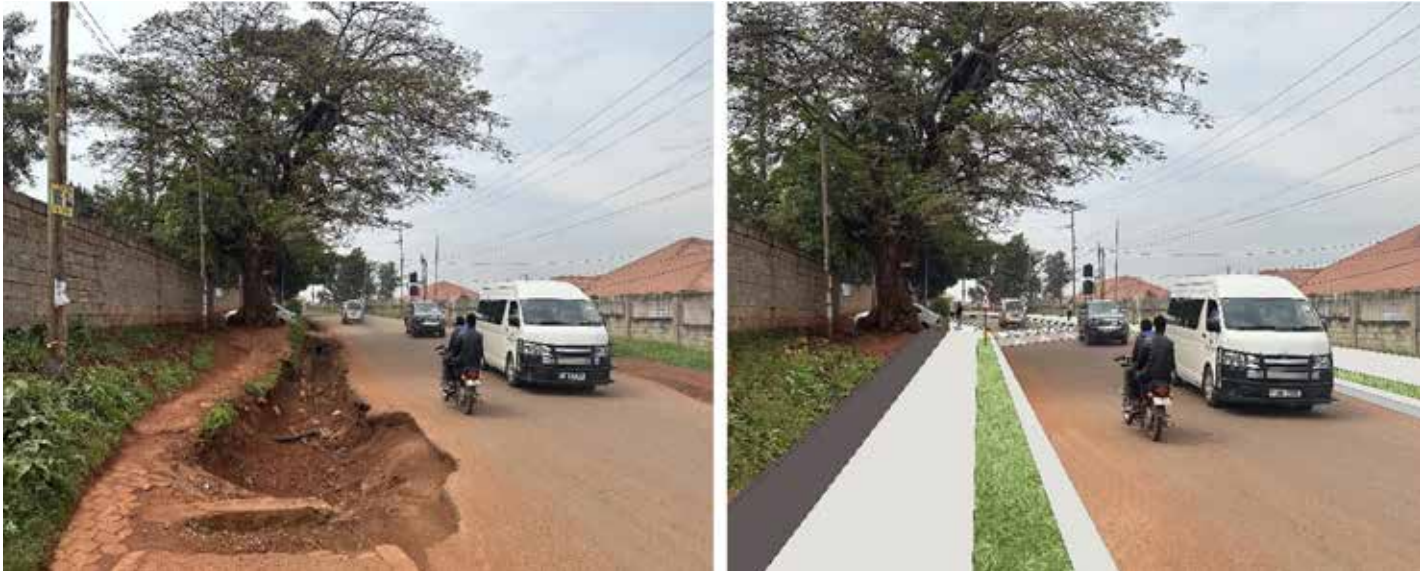
Robert Mugabe Road in front of Mbuya Church of Uganda primary school. Left- current situation; Right- proposed road diet and traffic calming intervention
