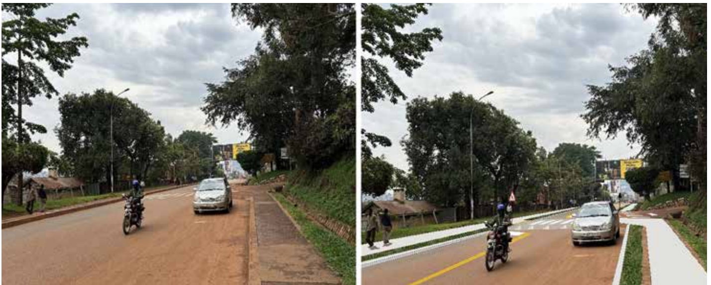
Gaba Road in front of St. Peter's primary school. Left- current situation; Right- proposed road diet and traffic calming intervention
