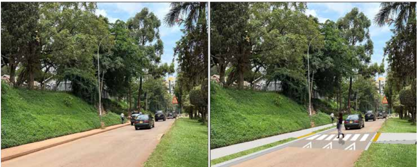
Lugogo Bypass near Kololo Senior Secondary school. Left- current situation; Right- proposed road diet and traffic calming intervention
