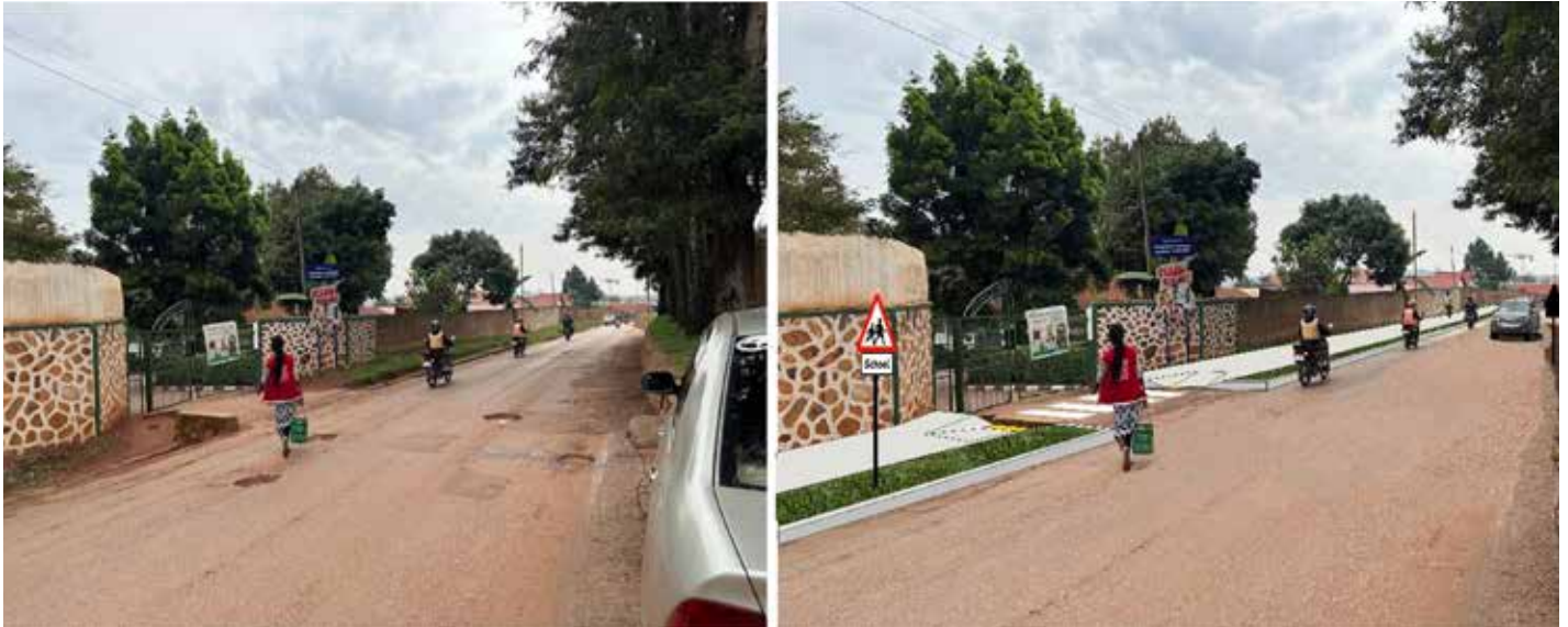
Nsambya Estate Road near St. Peter's primary school. Left- current situation; Right- proposed road diet intervention
