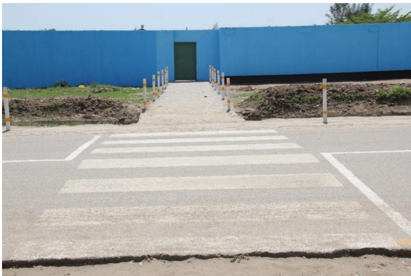
Figure 4. A new zebra crossing at the entrance of Kizito Primary School.
