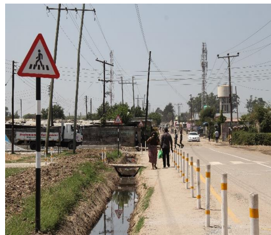
Figure 2. The Kizito Primary School before and after reconstruction. New reflected bollards are separating pedestrians from vehicles. The school premises are to the left-hand side Photo: Somela Sinkala.
