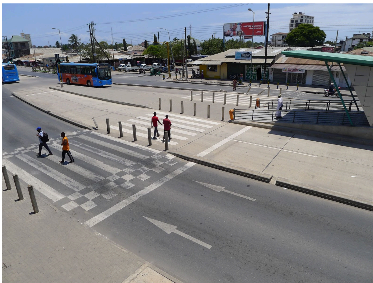
Figure 4. Safe crosswalk in Dar Es Salaam. (Institute for Transportation & Development Policy & United Nations Human Settlements Programme, 2022)
